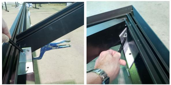
Drill access hole into Regular Rafter at Base thru clip or alternate drill into Hip Rafter
