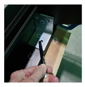
There are several locations where electrical from rough-in can be brought into Skylight at wood curb. (3 locations shown to drill thru frame base or curb)
