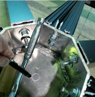
Drill hole thru Compression Ring into Rafter end-plate, then drill access hole / mount lamp hardware as needed in insure proper and safe attachment of fixture.
