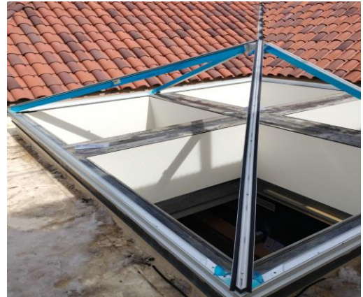
COMPRESSION RING & RAFTER Assembly for Pyramid
