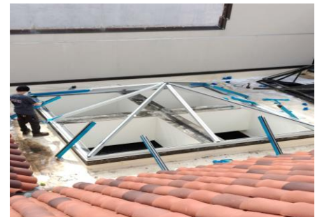
RAFTERS & HIPS to COMPRESSION RING Assembly (AKA Spider) for Structural Pyramid.
